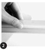
Press product into place on raceway. Join cables before placing next length.
